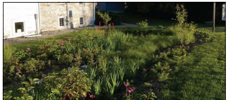
This raingarden designed by Land Works is located to catch runoff from a parking lot, to decrease stormwater impacts to the Otter Creek below.
